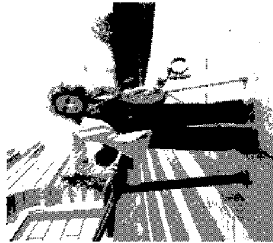
Handrails which do not project beyond the bottom tread are difficult for some who use them as a mobility aid. Projecting handrails also serve as a stair location cue for the visually impaired.
