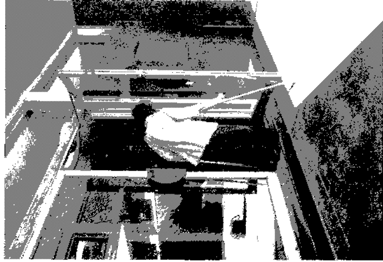
A step at the threshold is hazardous for all people but especially for those who use crutches. The door may close on the crutch and trap it.
