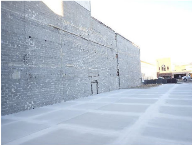
Figure 1. Overview of north end of east elevation.
