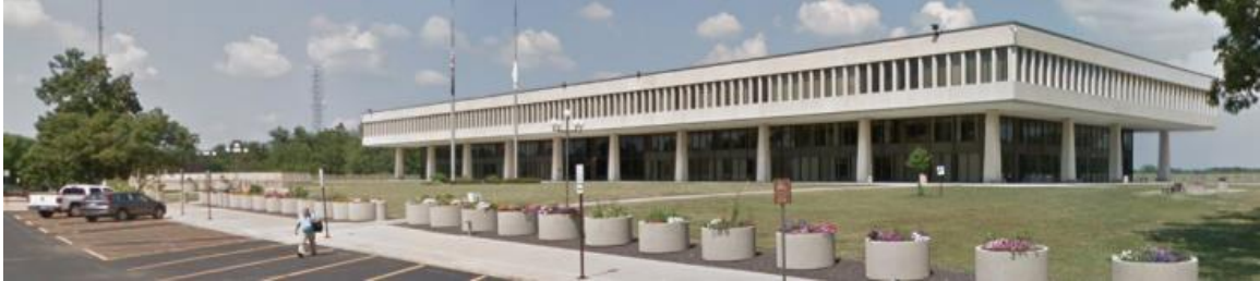
Existing Hanley Building
