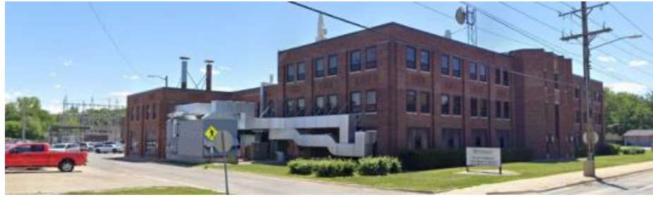
126 East Ash Street – Existing D6 & CBM Lab Facilities
