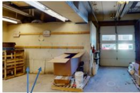
Concrete Interior shut-out panels
