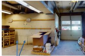
Concrete Interior shut-out panels
