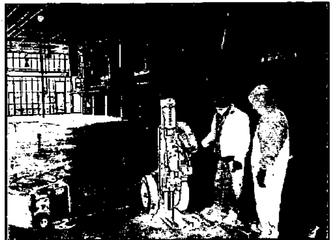
View of the location of boring B-202 in building SB-109.
