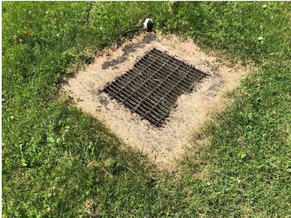
Photo 10: Drain identified on southeastern portion of assessment area
