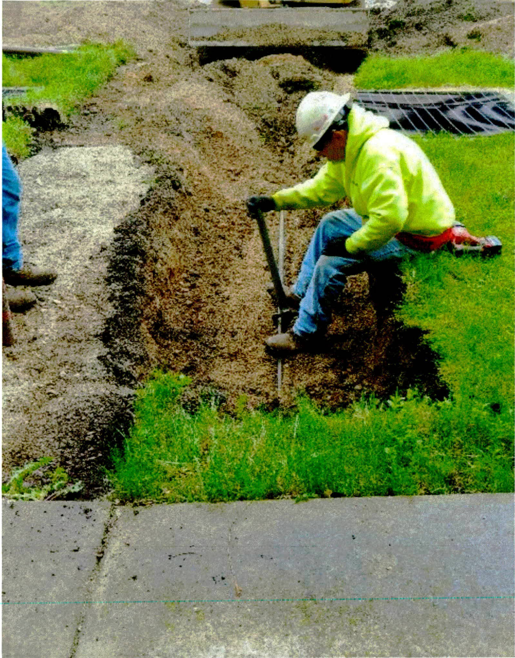
Photograph 13: View facing north of piping and vent line removal (May 17, 2019).
