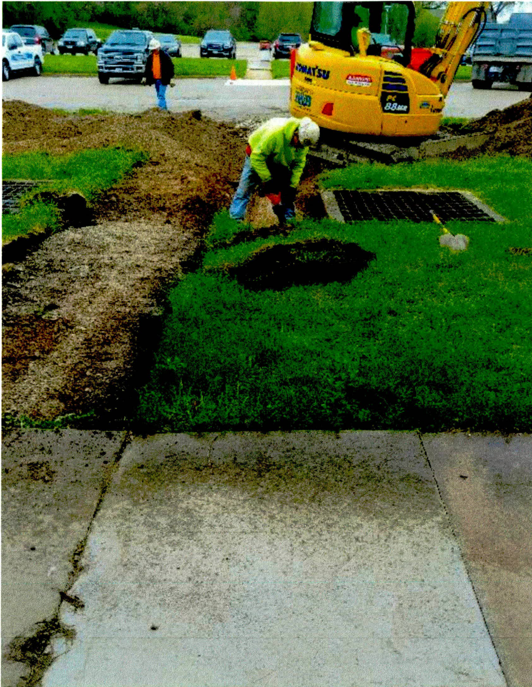
Photograph 12: View facing north of the vent and product line removal (May 17, 2019).
