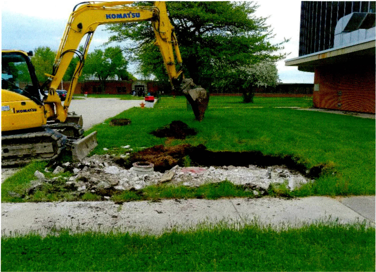
Photograph 1: View facing east showing the area of the UST (May 17, 2019).
