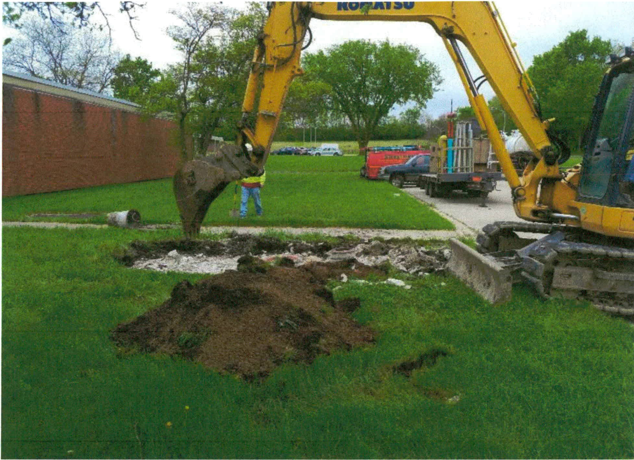
Photograph 3: View facing west showing the area of the UST (May 17, 2019).
