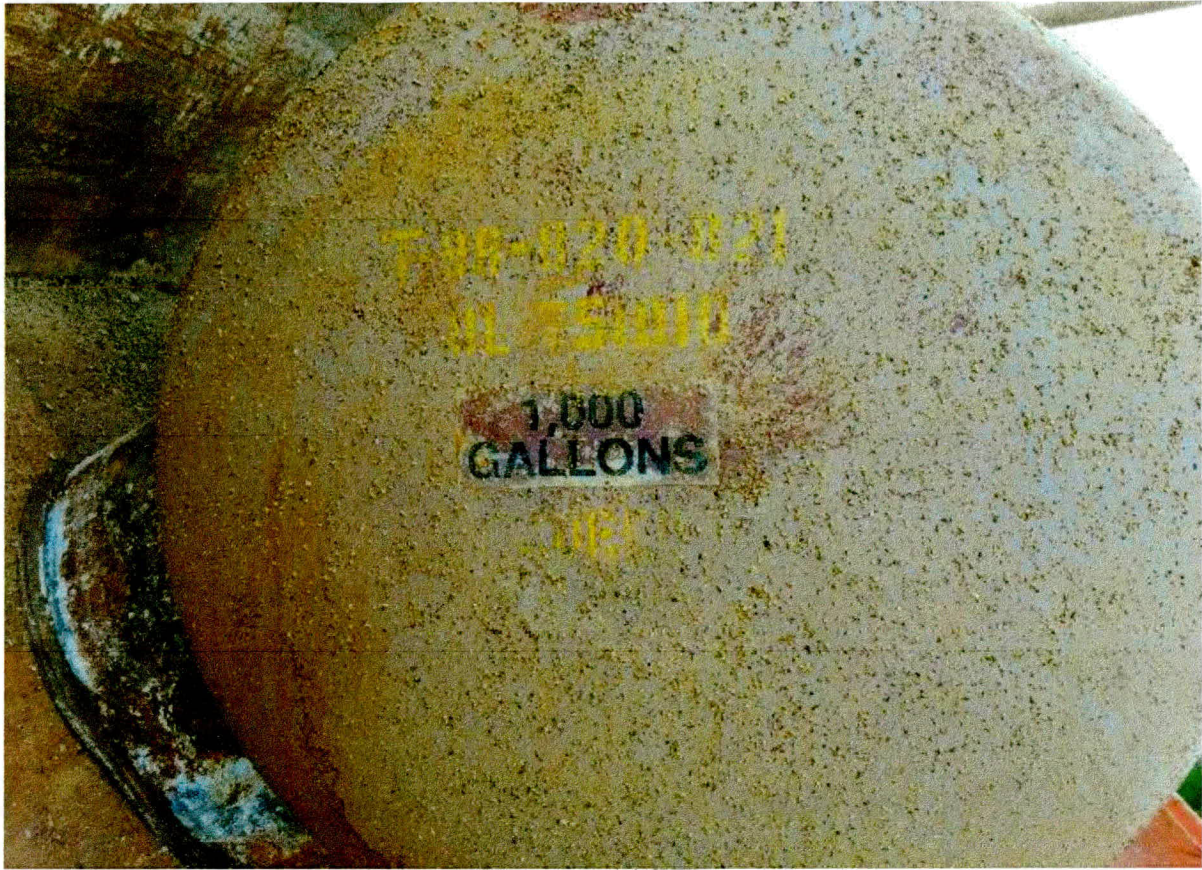
Photograph 10: View of 1,000-gallon fiberglass UST removed from the excavation and placed for transportation to disposal facility (May 17, 2019).
