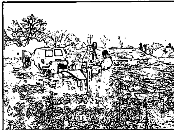
View of the location of boring B-203 in the location of former building SB-49.
