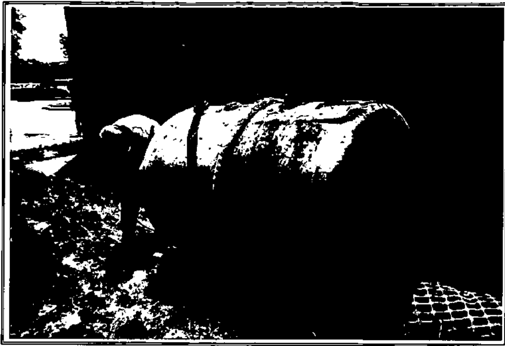
550-gallon diesel UST removed from the Chiller House excavation area. Fiberglass tank appeared to be in good condition and did not have any holes. Tank was cleaned and hauled off-site for disposal.
