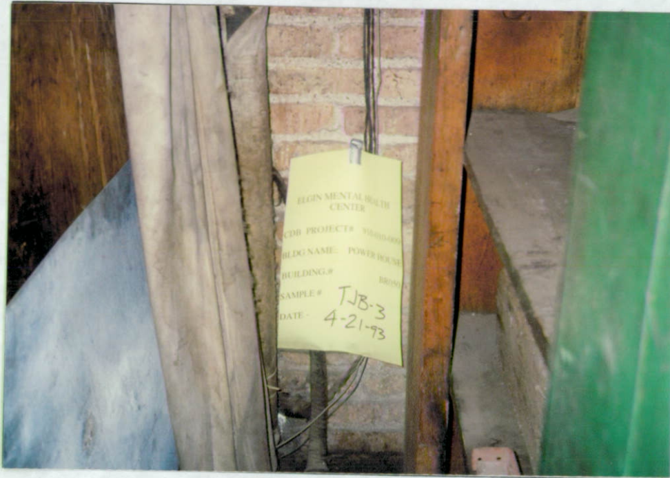
BR050-TJB-3 CEMENTITIOUS JOINT INSULATION ON PAPER WRAP PIPES
