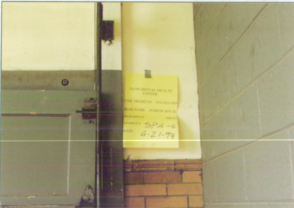
BR050-SPA-4 HARD PLASTER (PRE-1952)
