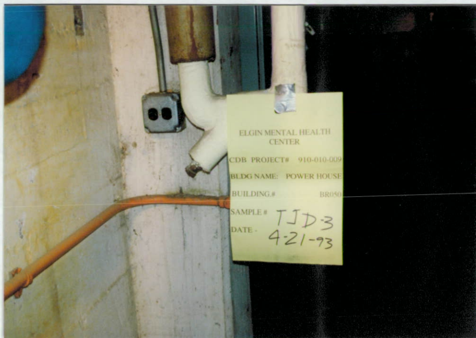
BR050-TJD-3 CEMENTITIOUS JOINT INSULATION ON FIBERGLASS PIPES
