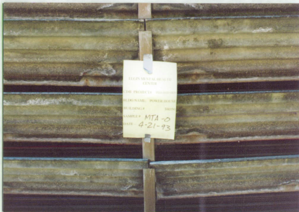
BR050-MTA-0 TRANSITE PANELS (ASSUMED)
