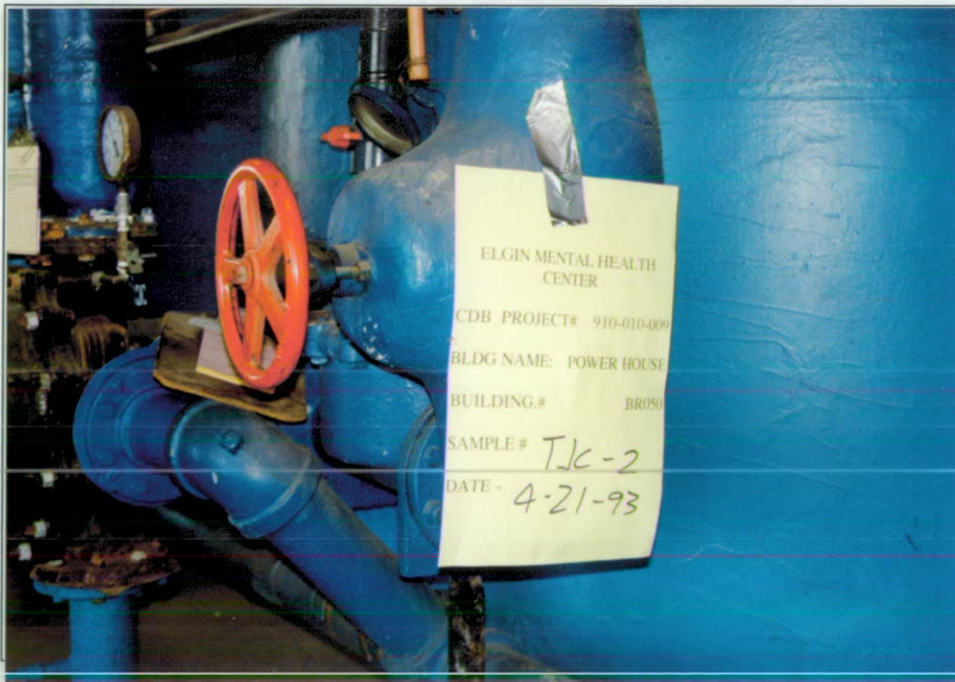
BR050-TJC-2 CEMENTITIOUS JOINT INSULATION ON AIRCCELL PIPES
