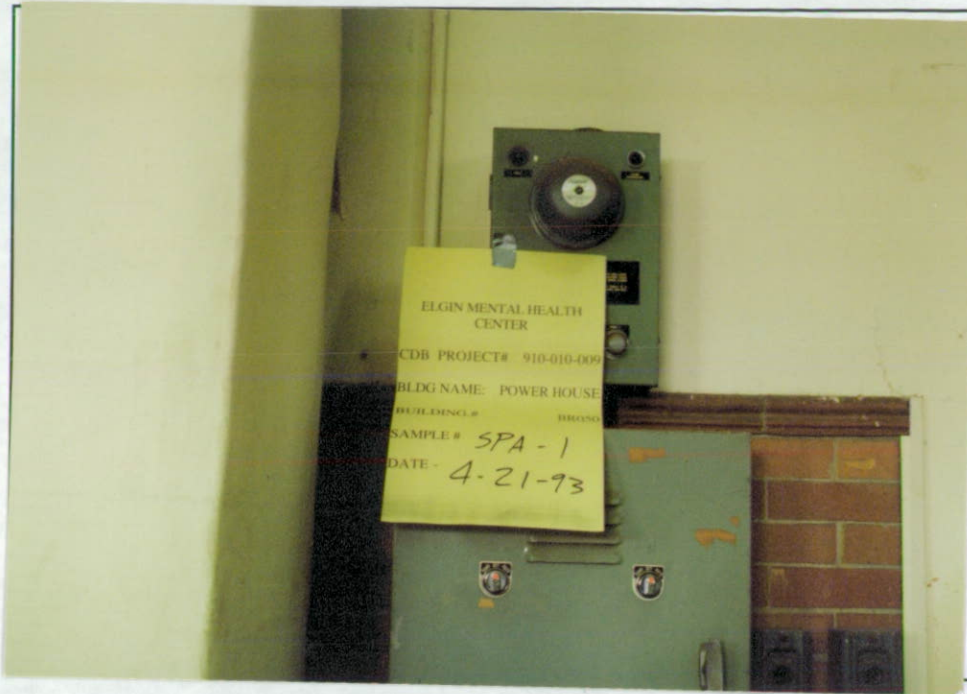
BR050-SPA-1 HARD PLASTER (PRE-1952)
