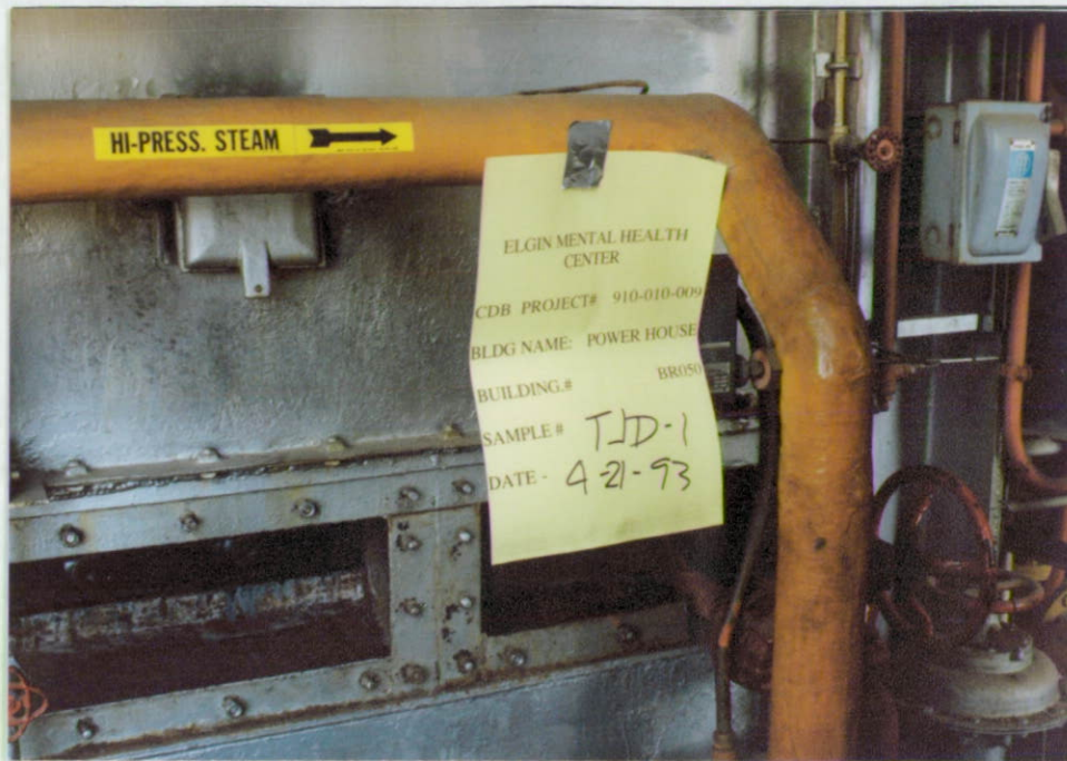
BR050-TJD-1 CEMENTITIOUS JOINT INSULATION ON FIBERGLASS PIPES
