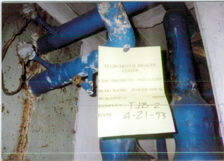
BR050-TJB-2 CEMENTITIOUS JOINT INSULATION ON PAPER WRAP PIPES
