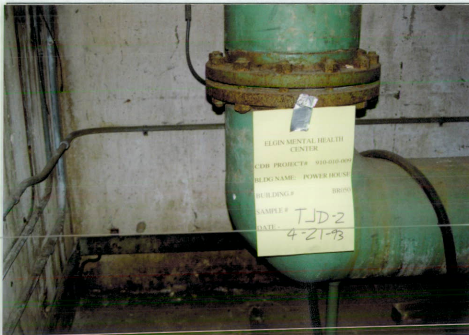
BR050-TJD-2 CEMENTITIOUS JOINT INSULATION ON FIBERGLASS PIPES
