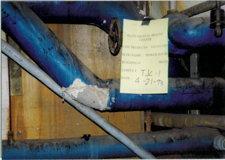
BR050-TJC-1 CEMENTITIOUS JOINT INSULATION ON AIRCCELL PIPES
