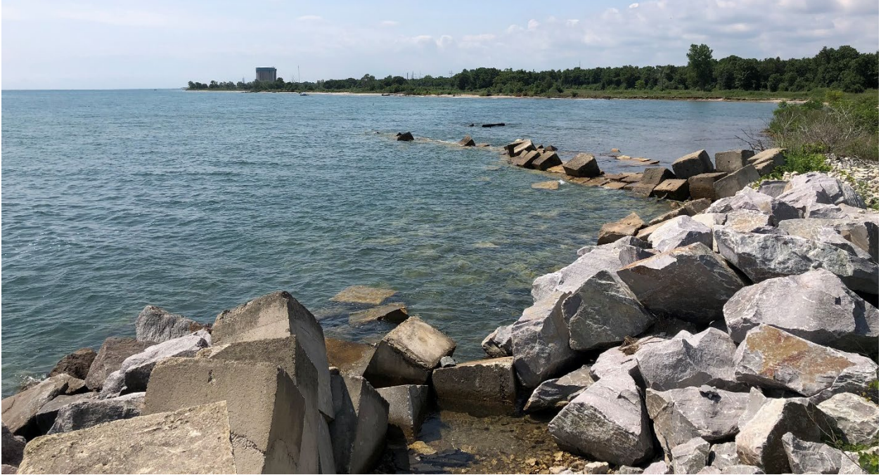
Figure 32: Concrete Blocks Located in Area 2
