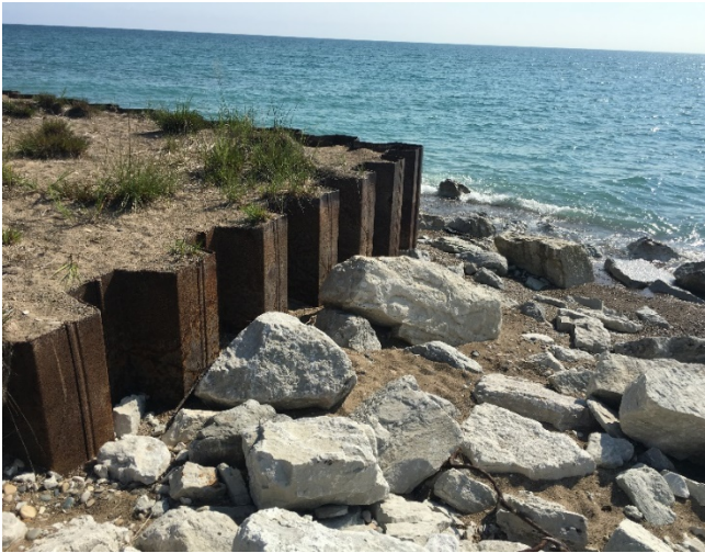
Figure 5: Sheetpile seawall along the resort and conference center
