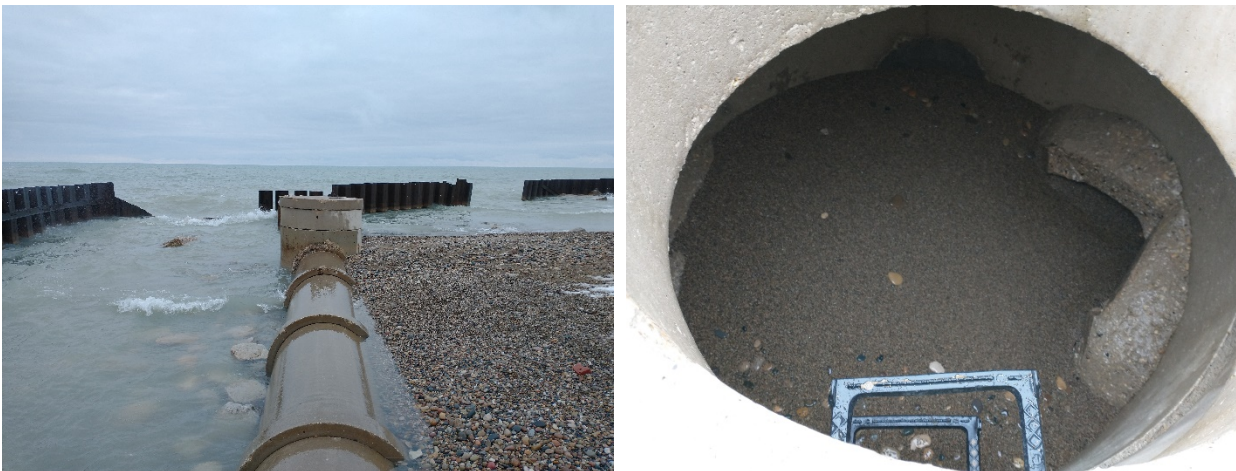
Figure 15: Stormwater Outfall Structure in Area 1 (photo taken 1/7/2021)
