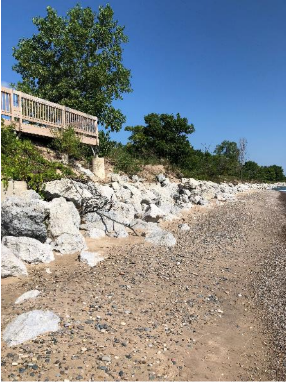
Figure E-11 Concrete Block & Rubble, ST 207+00 Looking North
