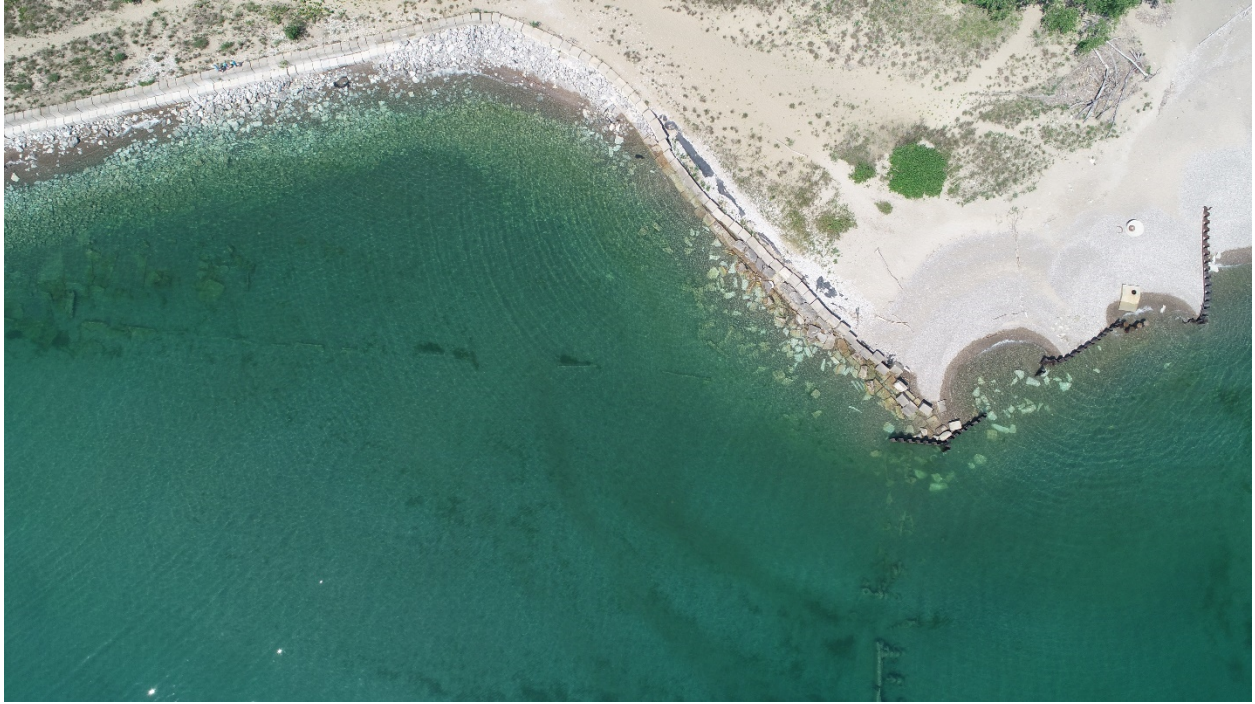
Figure F-5: Erosion behind sheetpile ST42+50 plan view
