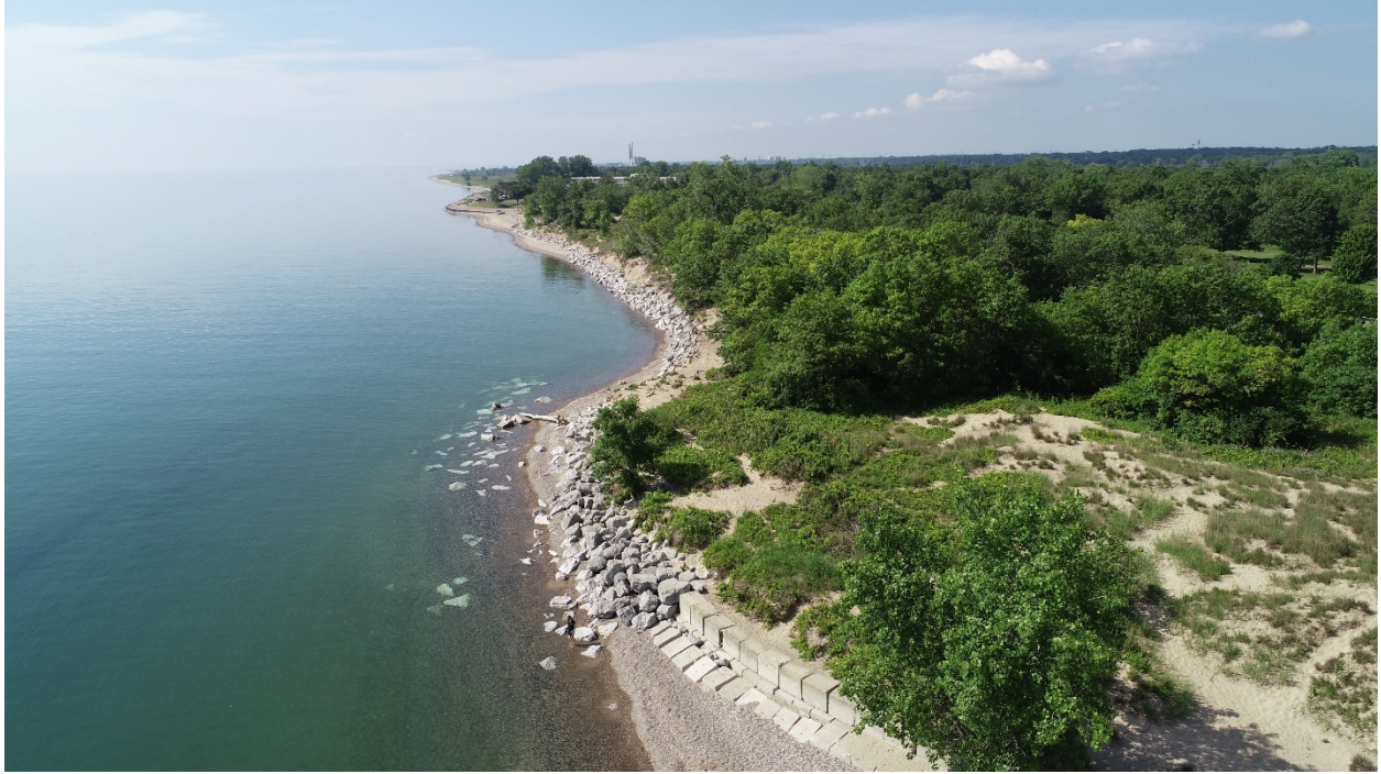
Figure F-11: Eco-block and riprap intersection at ST194+50 Looking South
