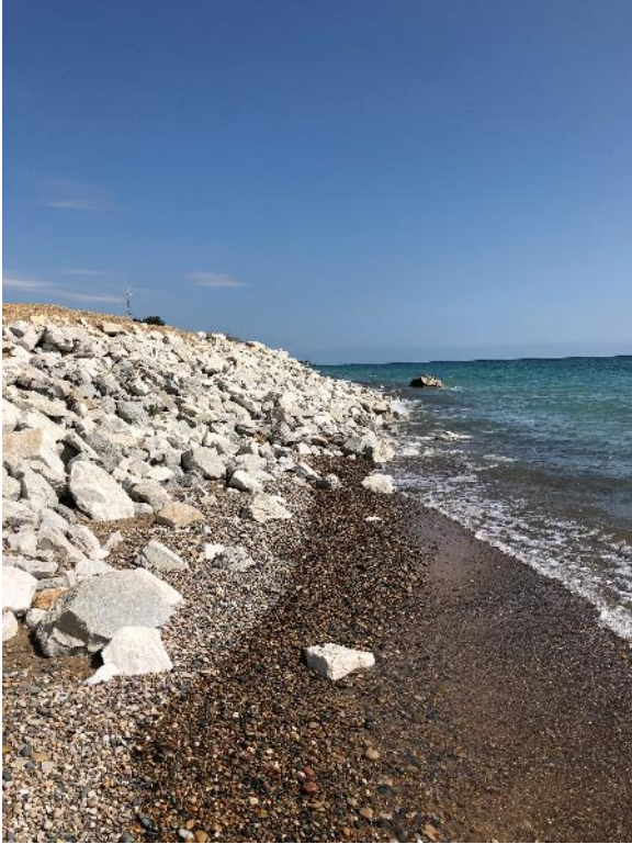
Figure E-7 Rubble Revetment, ST 185+50 Looking North
