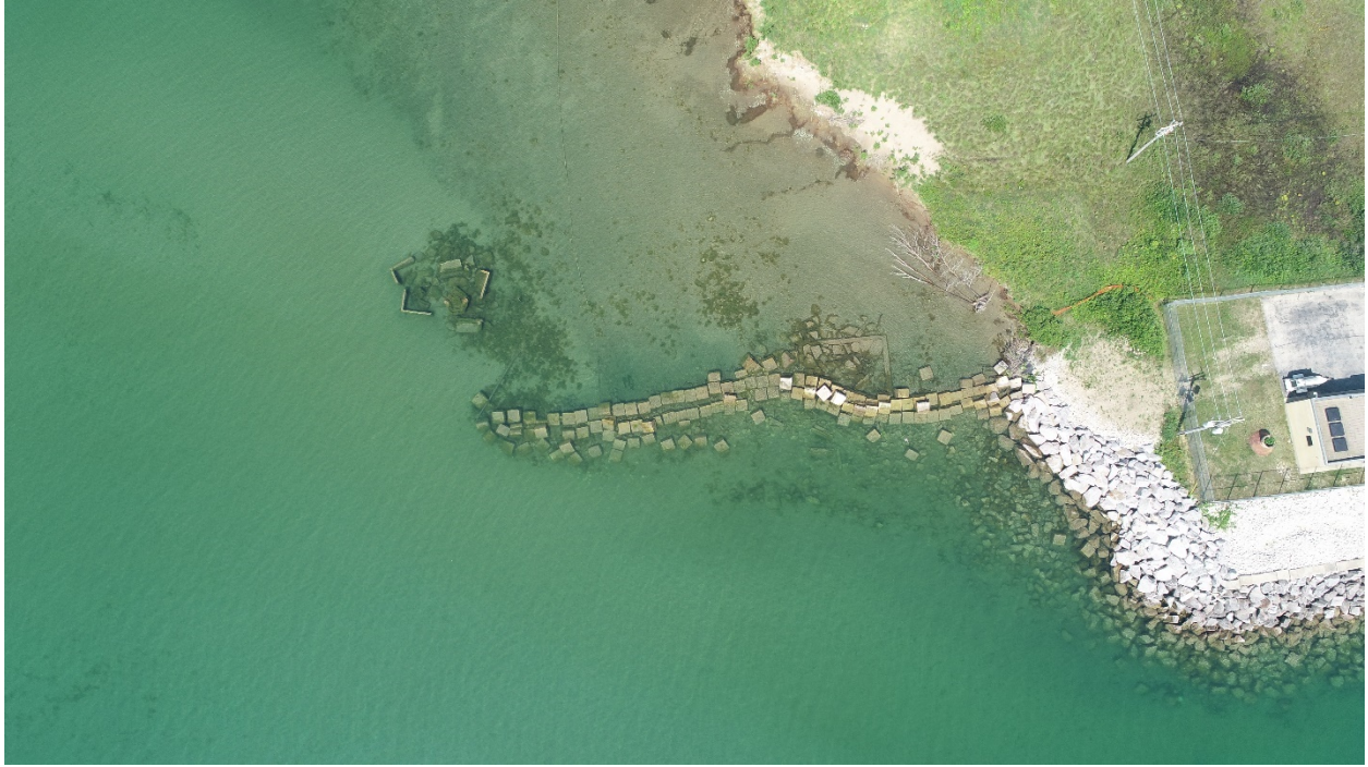
Figure F-9: Erosion at Area 2 ST 71+00 plan view
