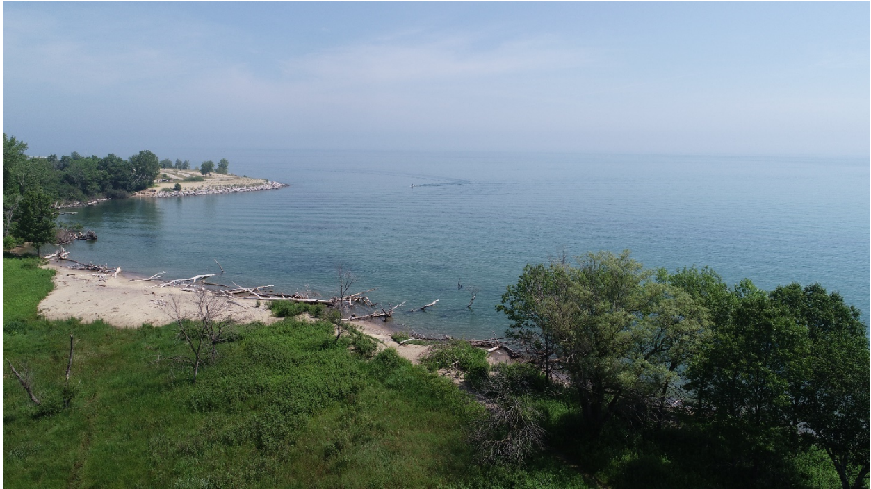
Figure F-2: Area 1 Northpoint marina breakwater. ST 15+00 Looking Northeast
