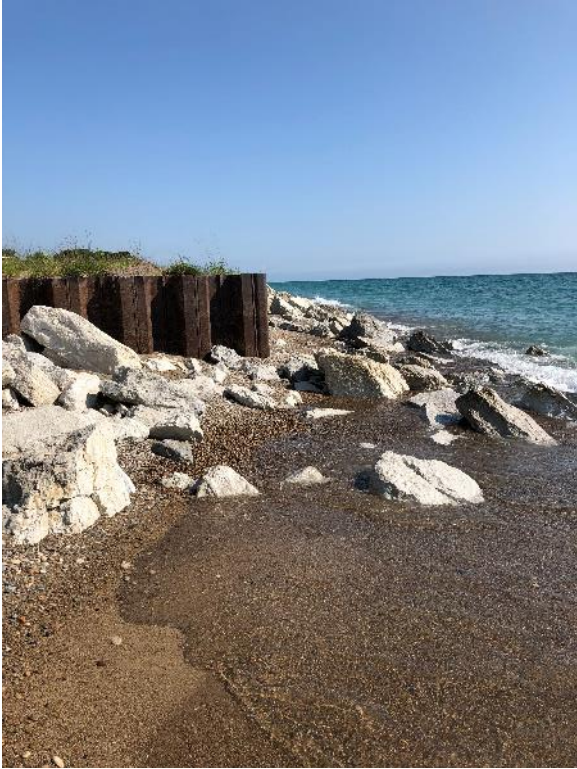
Figure E-16 End of Sheetpile Wall, ST 222+00 Looking North
