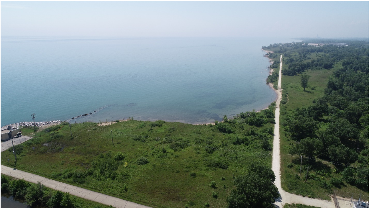
Figure F-8: Erosion at Area 2 ST 71+00 Looking South
