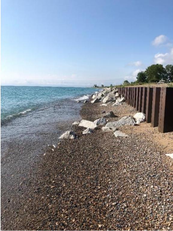
Figure E-15 Sheetpile Shoreline, ST 214+00 Looking South
