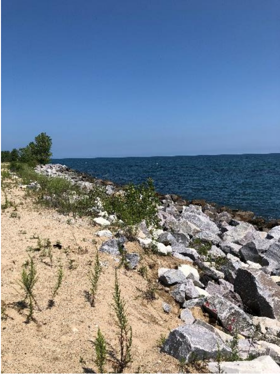
Figure E-1 Riprap Revetment, ST11+00 Looking North
