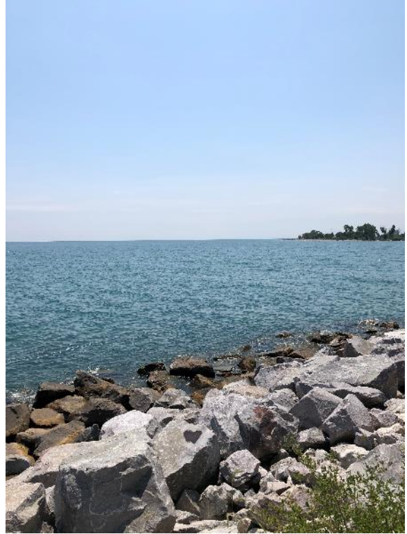
Figure E-2 Riprap Revetment, ST11+50 Looking South
