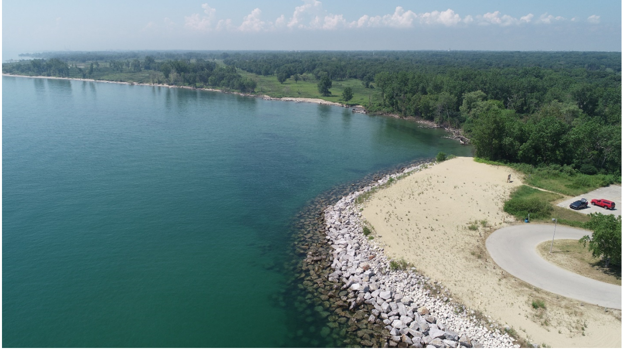
Figure F-1: Area 1 Northpoint marina breakwater. ST12+50 Looking Southwest
