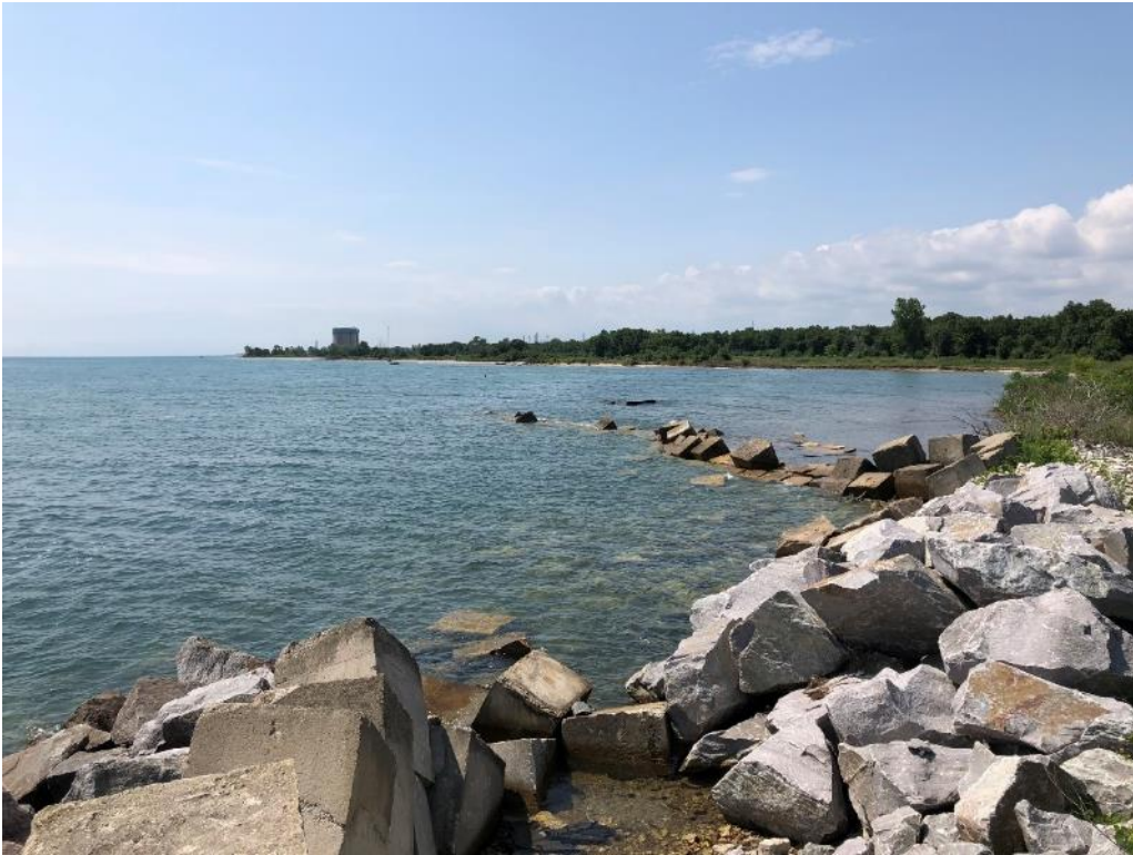
Figure E-5 Southern End of Failing Block & Rubble Revetment, ST71+00 Looking Southwest
