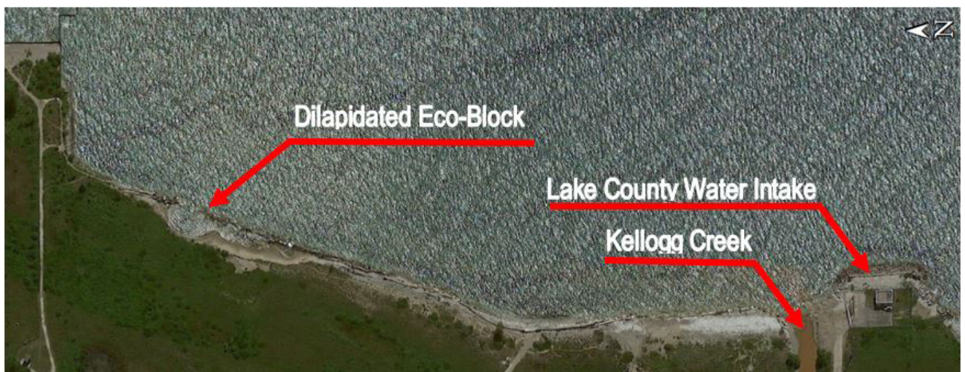
Figure 26: Damage and erosion of the shoreline north of the Lake County water intake station, (map data: Google, TerraMetrics)
