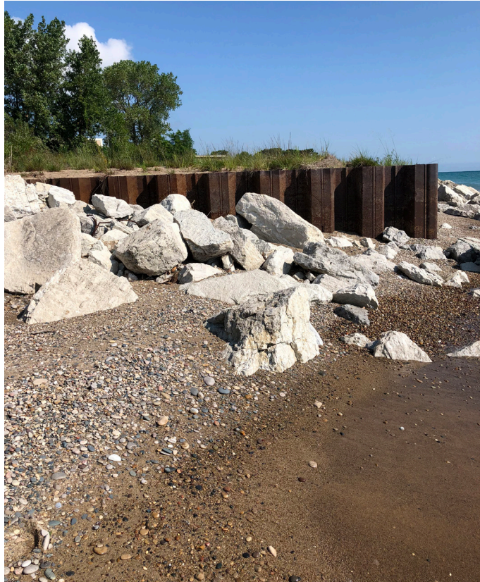
Figure 33: Sheetpile seawall along convention center
