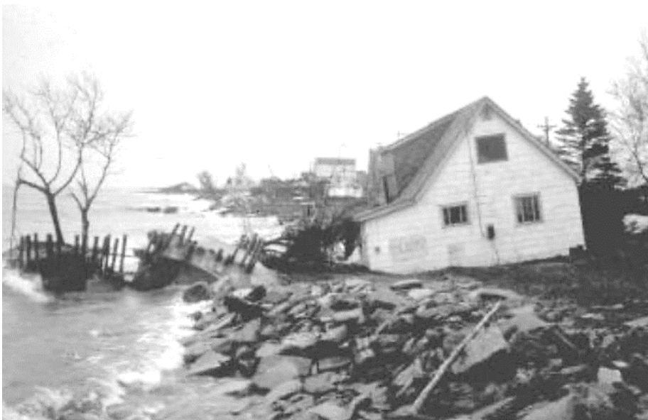
Figure 5: Severe erosion within the North Unit (photo by Illinois State Geological Survey, April 1973)
