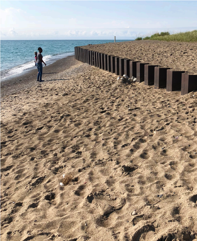
Figure 32: Steel sheetpile across recreational beach
