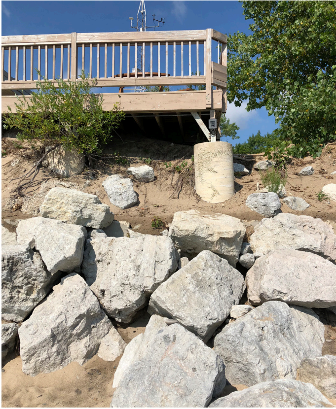
Figure 31: Exposed footing and riprap placed in front of the park office
