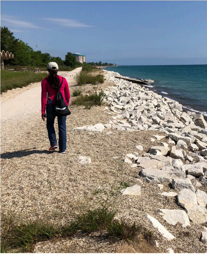
Figure 30: Riprap placed to protect the sidewalk north of the Swimming Beach.
