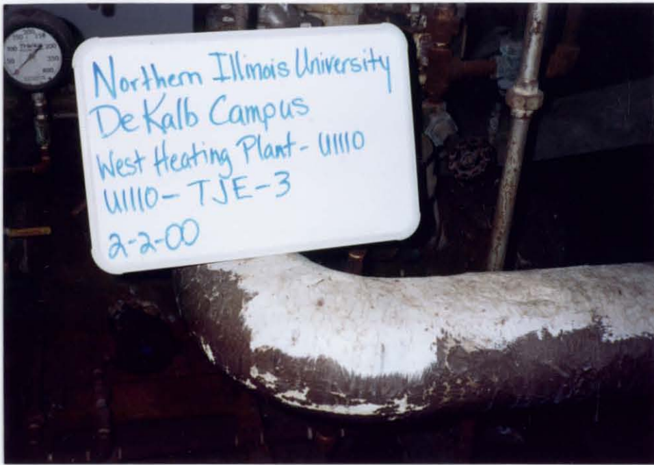
U1110 - TJE - 3 FITTINGS ON MAG-BLOCK PIPE INSULATION (ADDITION #1 - 1964)
