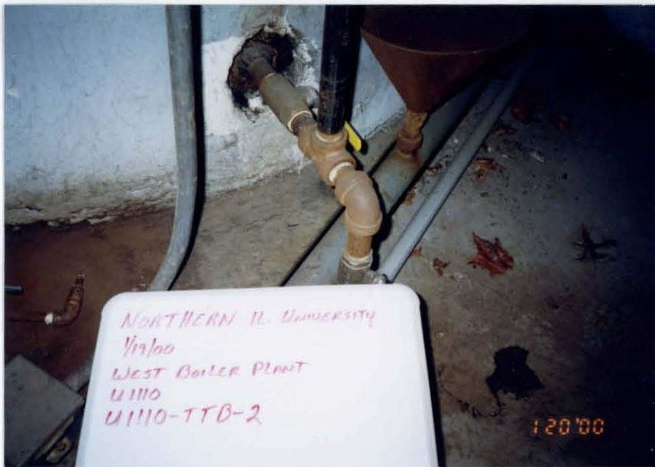
U1110 - TTB - 2 RECEIVER TANK INSULATION (ADDITION #1 - 1964)
