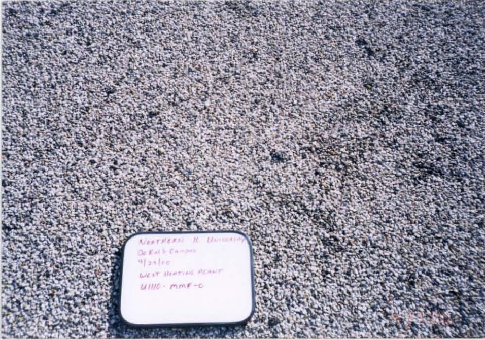
U1110 - MMF - 0 BUILT-UP ROOF (Addition #1 - 1964)
