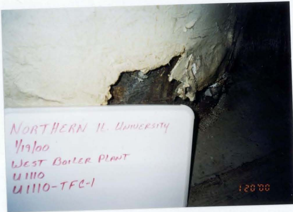
U1110 - TFB - 1 BOILER STACK INSULATION ON BOILER #3 (ADDITION #1 - 1964) (Picture is incorrect. Material designation was changed to TFB.)
