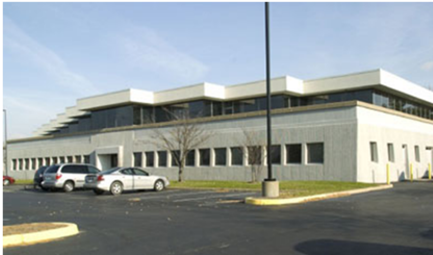
Building 200: A two-story building comprised mainly of concrete with a ribbed finish and a characteristic sawtooth roofline for the second story.
