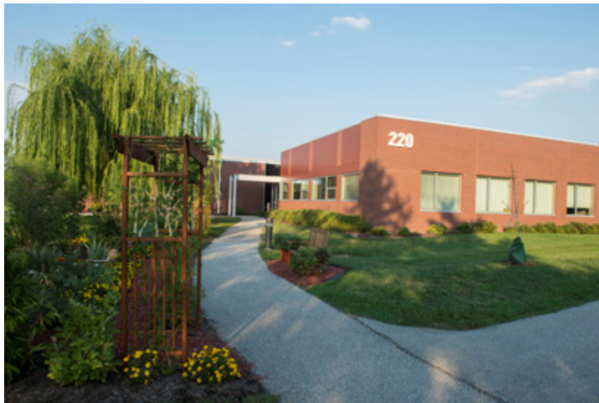
Building 220: A one-story building comprised of a combination of brick and Trespa panel.
