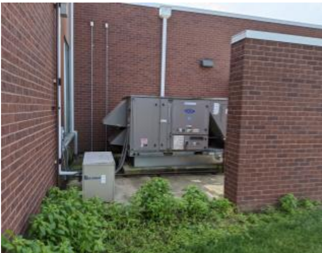
Photo 27 Air handling unit for building 220
