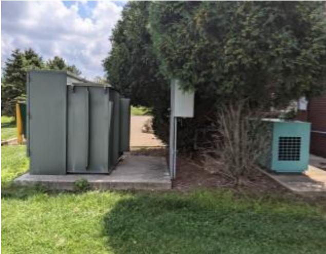
Photo 25 Transformer and emergency generator
