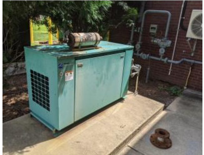
Photo 26 Emergency generator for building 220
