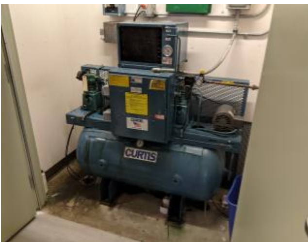
Photo 41 Air Compressor in building 220
