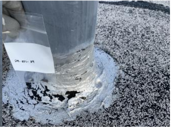
Photo 30: HA 29, black tar with silver paint located around the base of vents and HVAC on the main roof.
