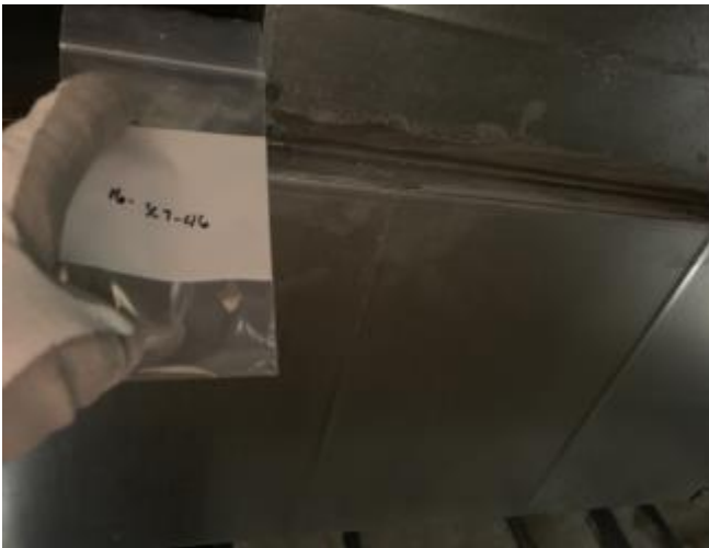
Photo 17: HA 16, grey duct sealant on the HVAC seams.
