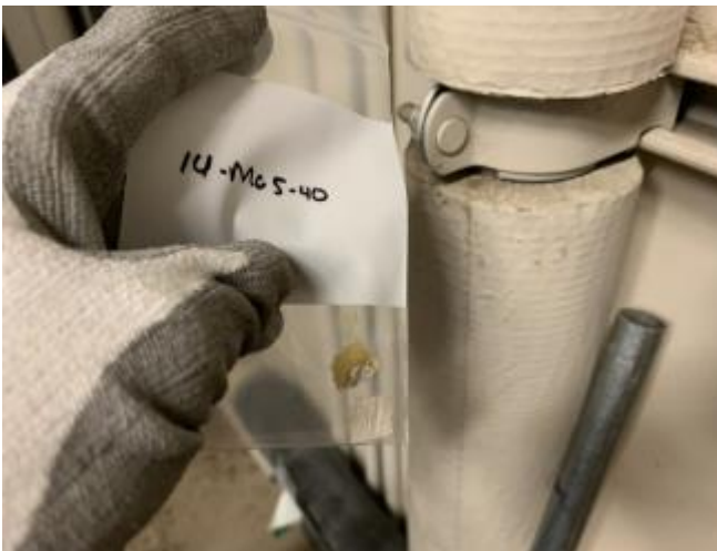
Photo 15: HA 14, white pipe end mastic located in the mechanical room and hallways.
