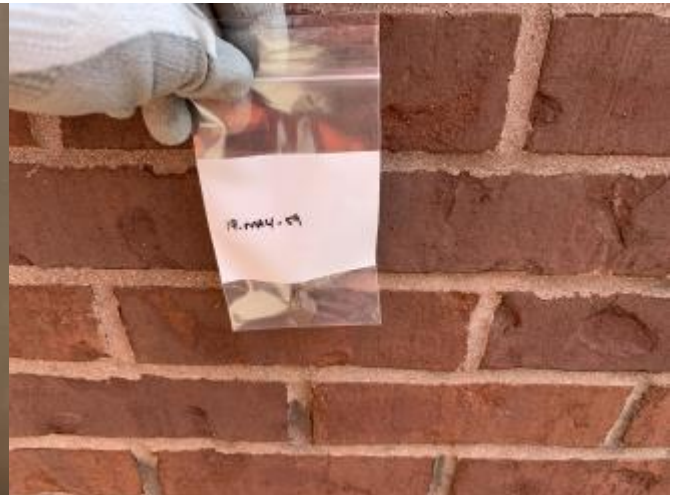
Photo 20: HA 19, brick grout located on the exterior.
