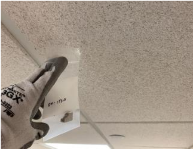
Photo 5: HA 04, 2' x 2' rough textured ceiling tiles located in the office areas.
