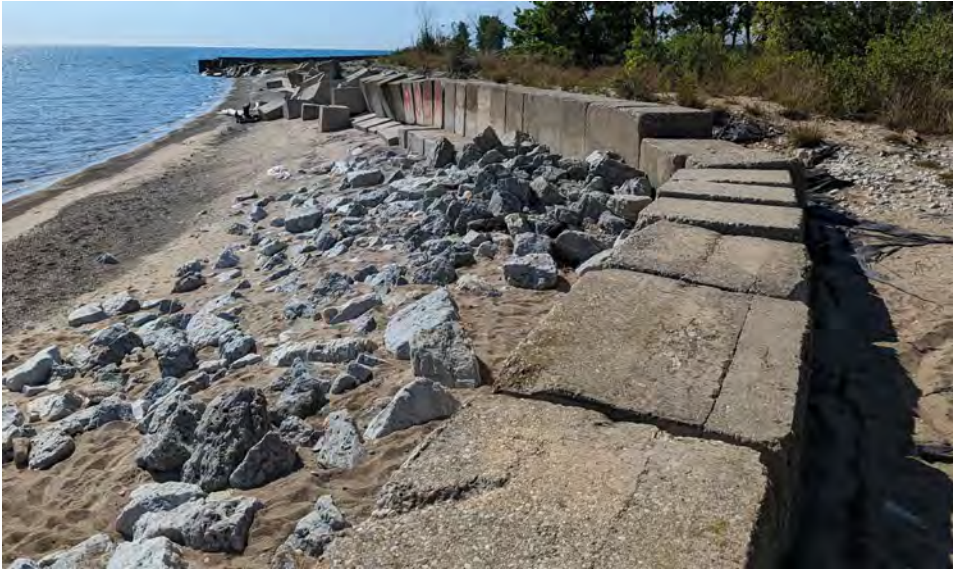
SALVAGED CONCRETE ECO BLOCKS
